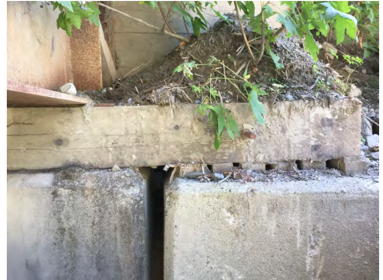
Down stream left abutment shim
