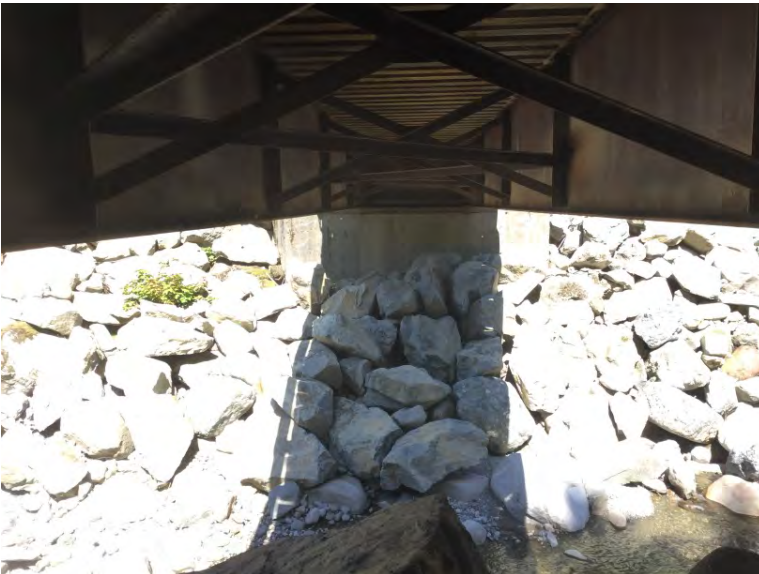
Right Bank Abutment when facing downstream
