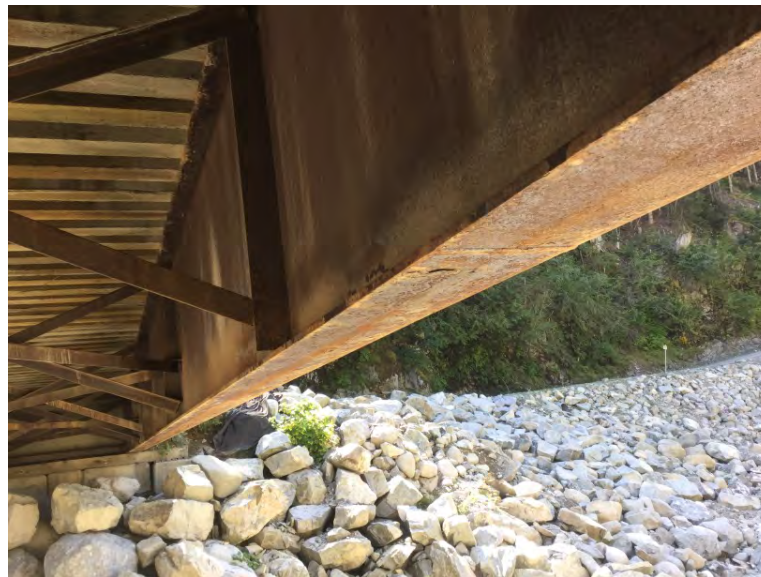
Corrosion
