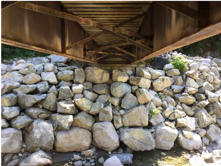
Left Bank Abutment when facing downstream
