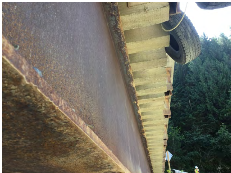
Timber deck to girder connection
